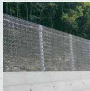
落石防護柵工 E-FENCE
