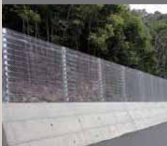
落石防護柵工 E-FENCE
