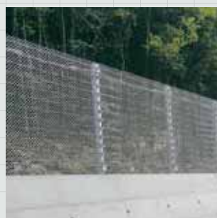
落石防護柵工 E-FENCE
